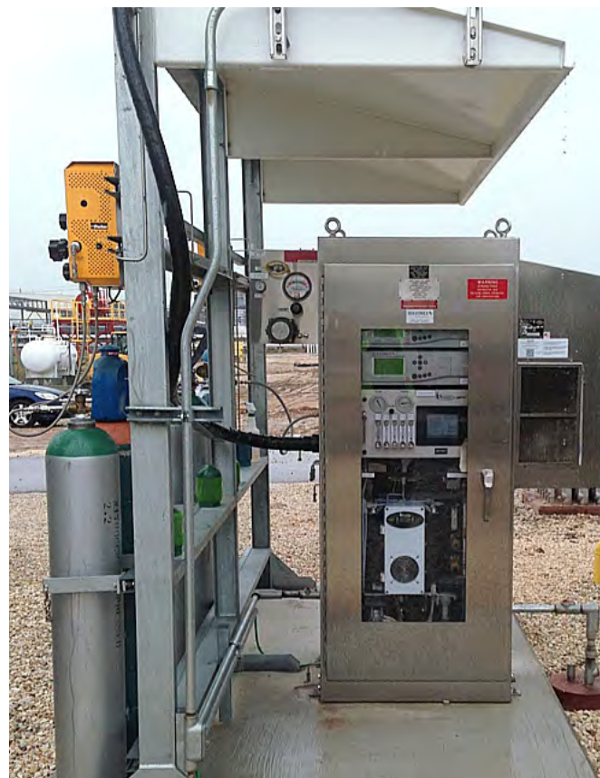
A multi-gas monitoring system in a protective outdoor enclosure.
