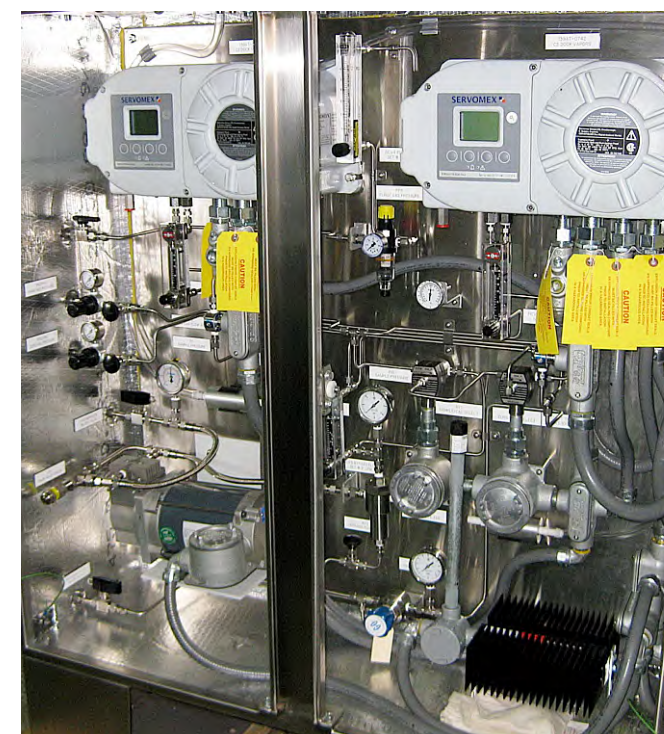
A redundant oxygen monitoring system, based on two SERVOTOUGH Oxy 1900 analyzers.
