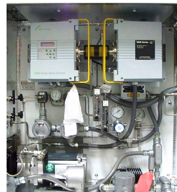
An emissions control system using the SERVOTOUGH SpectraExact 2500 Infrared analyzer to monitor hydrocarbons.
