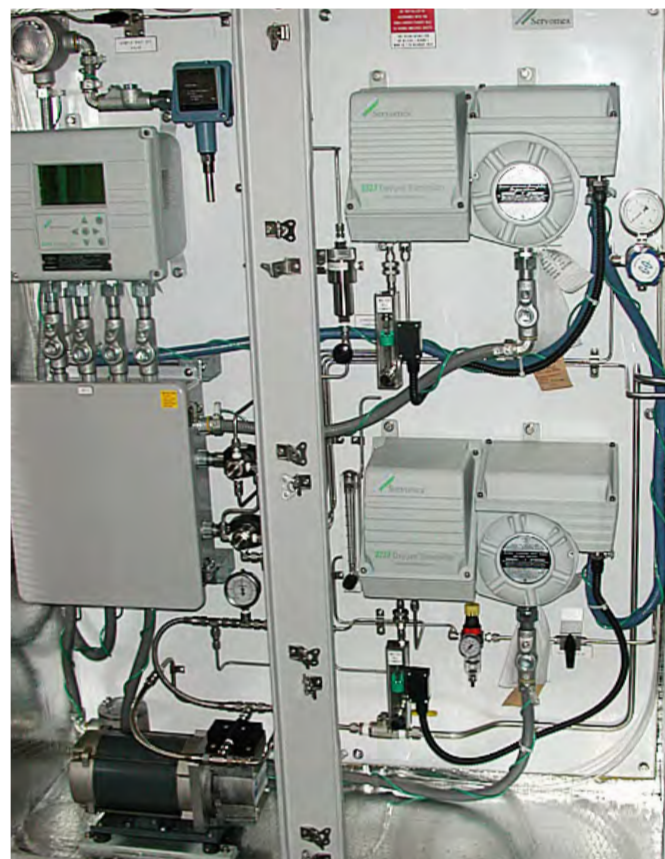
A redundant oxygen monitoring system, based on two SERVOTOUGH OxyExact 2200 analyzers.
